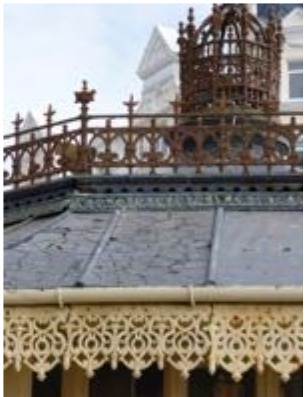
From top: the kiosk in about 1893 from the James Gray Collection; the kiosk today; roof and ironwork in poor condition
