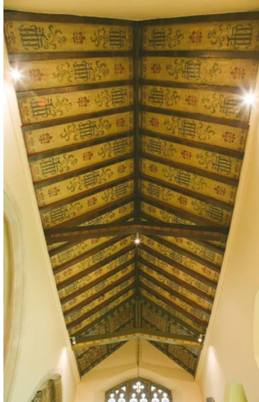
The restored ceiling to the Lady Chapel: this victorian work is stencil upon a lino-based material.
