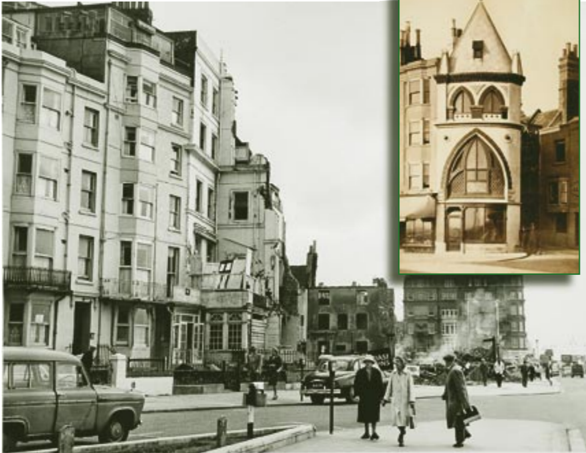
Two views of 67 Kings Road, Brighton: the building in the sepia image, photographed around 1870, was demolished in 1897, while the view above shows the 1963 clearance for the Brighton Centre redevelopment.
